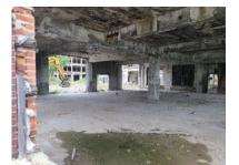
Interior of west end of plant. The narrow building width made it difficult to modernize for new automated assembly line machinery.
