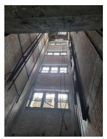
6-story elevator shaft for moving industrial materials and automobiles between floors of Packard plant.
