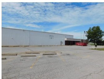
Cord production facility, 9620 E Broken Arrow Expressway
